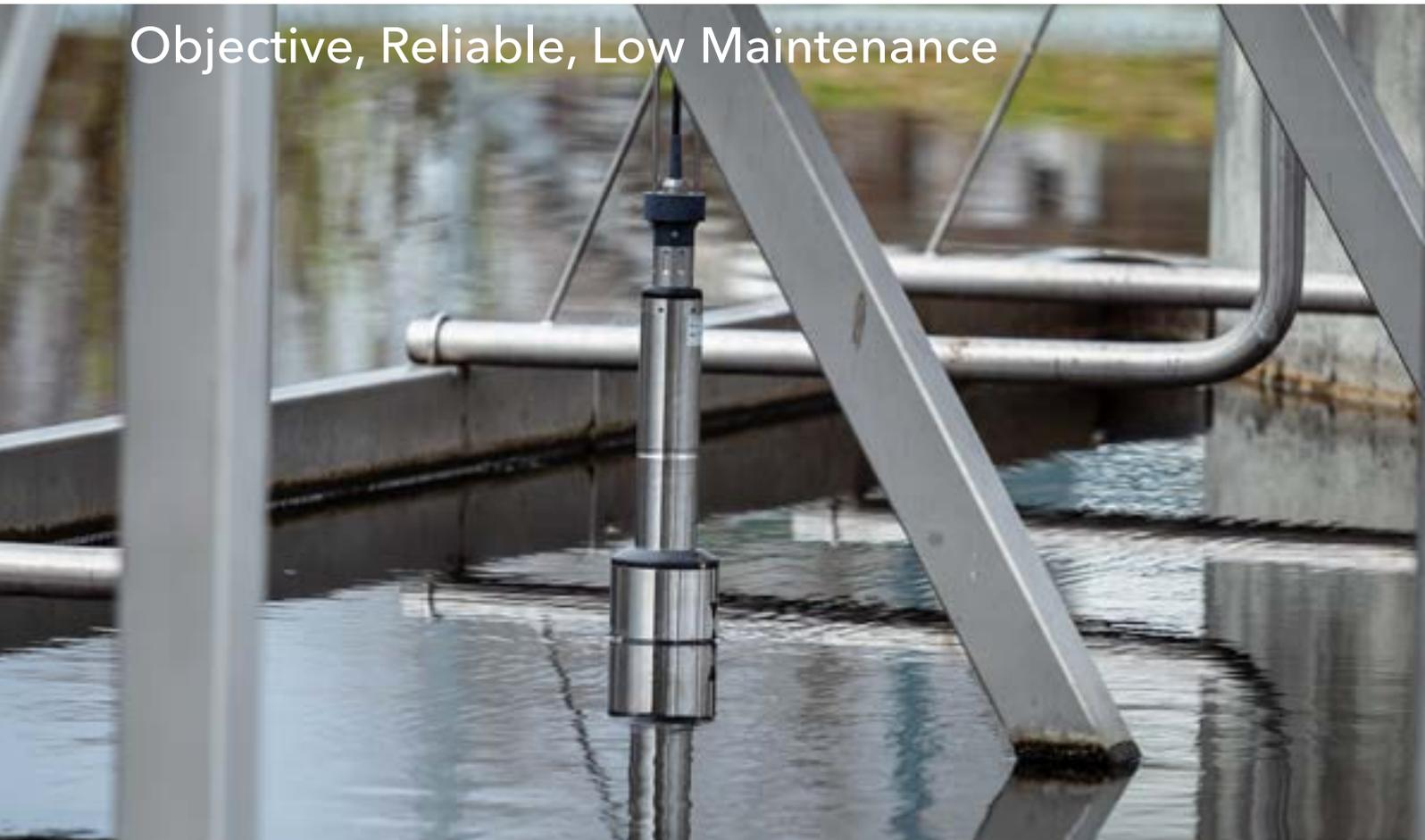
The sludge level is the boundary of settled sludge to the projecting turbid or clear water, wherein the location of the sludge level is defined as the distance to the water surface (sludge level depth), or as distance from the tank bottom (sludge level).
