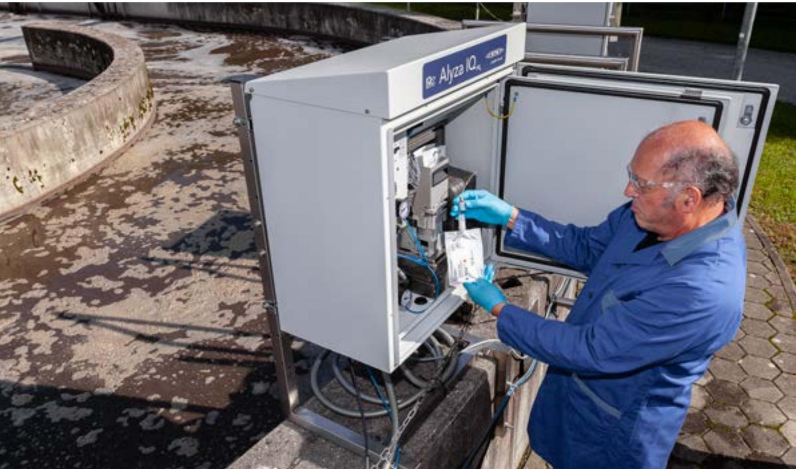
In the wastewater treatment industry, there has been an increased need for on-line measuring analyzers justifying their market presence next to less expensive in-situ sensor systems. Especially when it comes to high-precision water analyses, for example in the monitoring of the discharge in sewage treatment plants requiring automatic calibrations and/or adjustments as well as standard DIN methods for analysis, analyzers are necessary.
